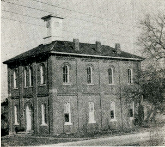
Methodist Church and Masonic Hall at Hermitage Used by both Methodist and Christian Churches
