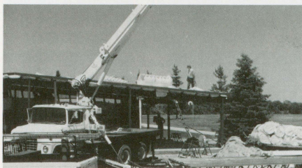
Roof insulation being applied.
