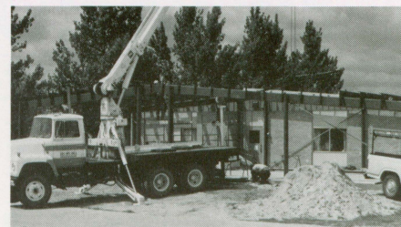
Hoisting the steel rafters.
